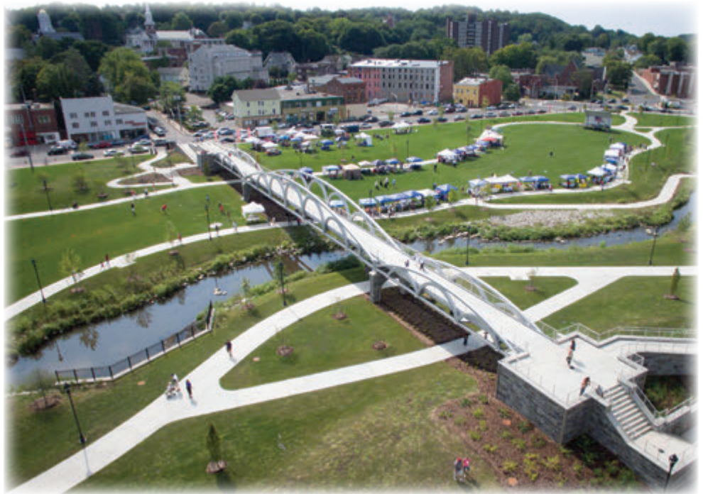
Above is an aerial view of Meriden Green & Silver City Bridge
